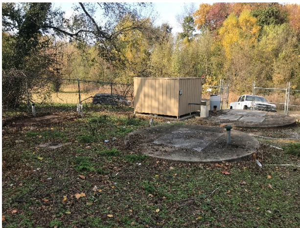
Simmons Lift Station Area
