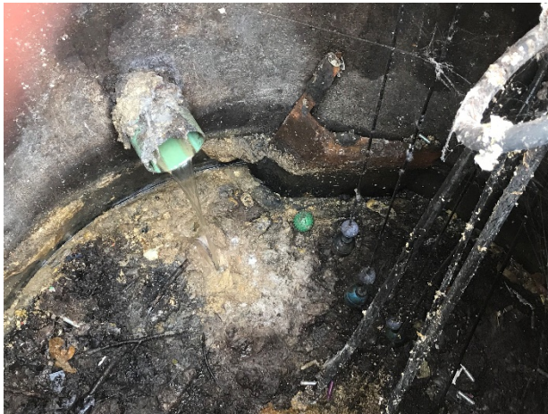
Maloree Plate in Wet Well
